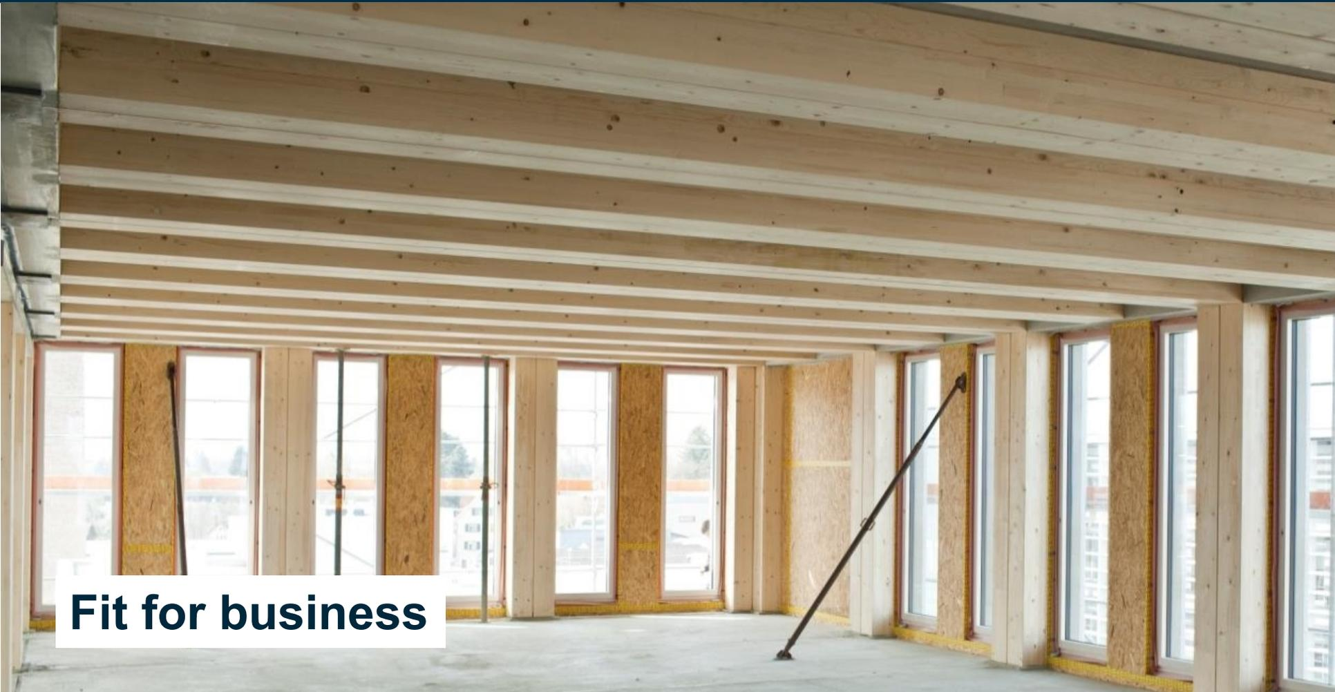
A wide-angle photograph of a building's interior during construction. The ceiling is composed of numerous parallel wooden beams. The walls are partially finished with vertical wooden studs and sections of oriented strand board (OSB). A series of windows runs along the back wall, with some sections still under construction. A long, thin metal rod or pipe is leaning against the wall on the right side. The floor is a smooth, light-colored concrete.
