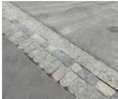
Granite cobbles are used to articulate the transition between different zones.
