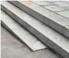
Existing stairs are retained, and new stairs are produced from similar granite.
