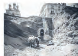
Excavations de la casemate 1915
