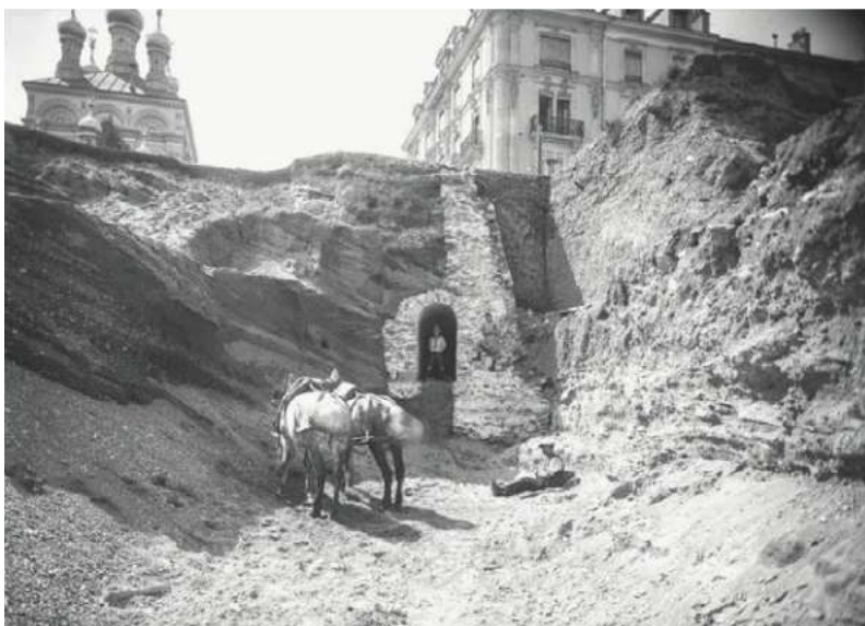
Excavations de la casemate 1915
