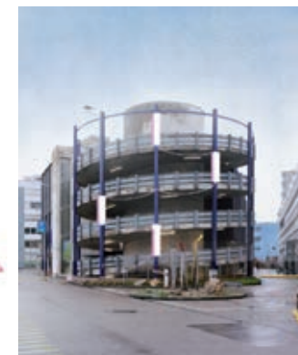
Filtration system on south facade
