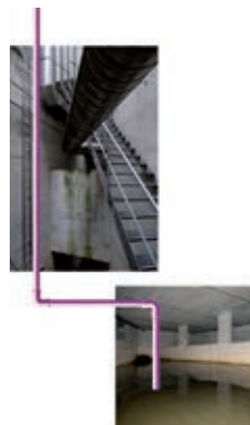
Pipes leading to the roof
