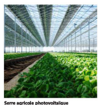
Serre agricole photovoltaïque
