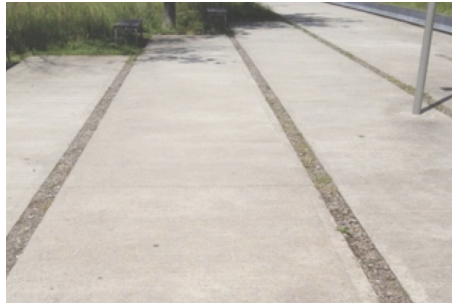
Joints large gravier / terre (route)
