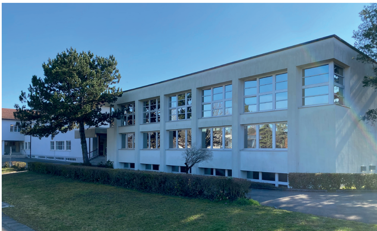
Trakt 3 Nord-West-Fassade Sporthallen
