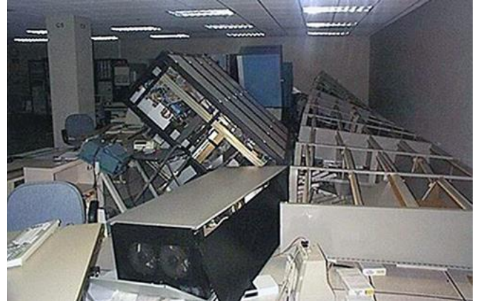
Abb. 2.21.2 > Umgekippte Computerracks
