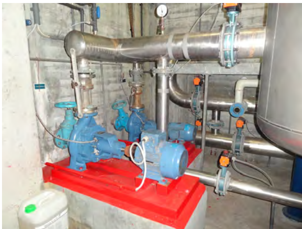
Filterpumpen
