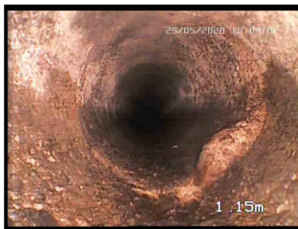
, 00:00:47, 1.14 Remarque générale / JOINT BETON APPARENT
