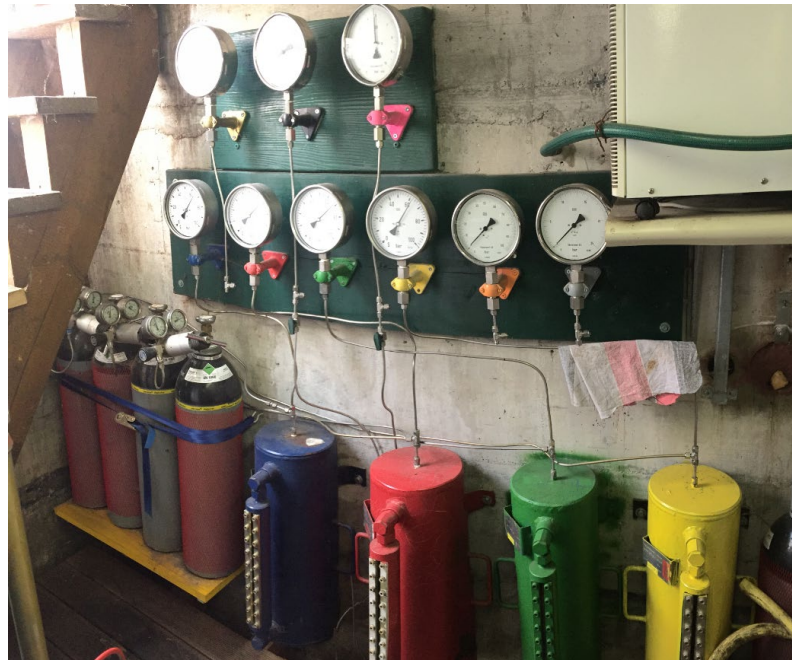
Figur 8: Packer-Pressure-Maintenance-System
