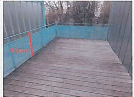
Photo 4 Garde-corps terrasses rez non conformes
