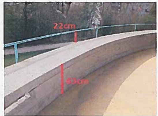
Photo 4 Garde-corps terrasses rez non conformes
