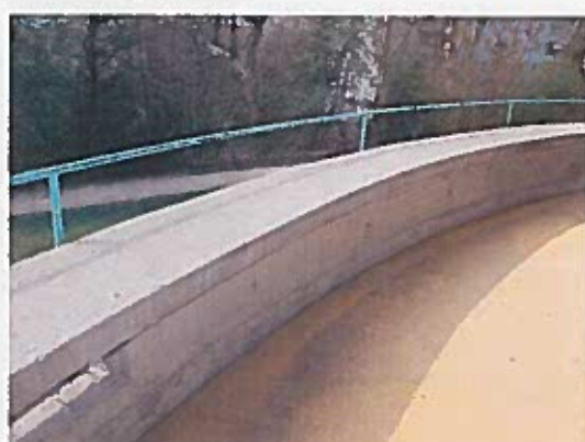
Photo 12 Garde-corps non conforme
