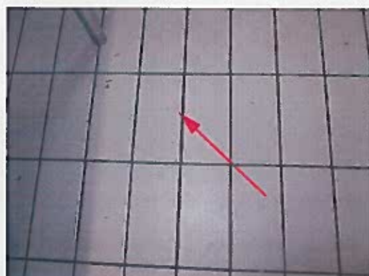
Photo 10 Fissures des carrelages
