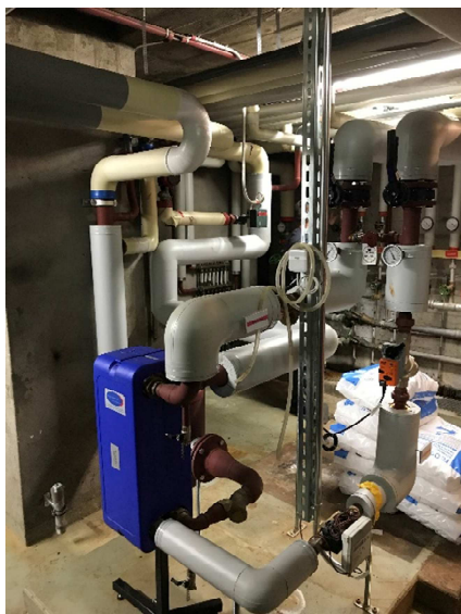
Figure 2 : Raccordement CAD
