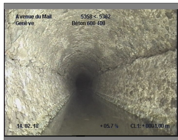
Photo: 17_17_153_A.JPG, 00:00:26 1m, Retenue d'eau
