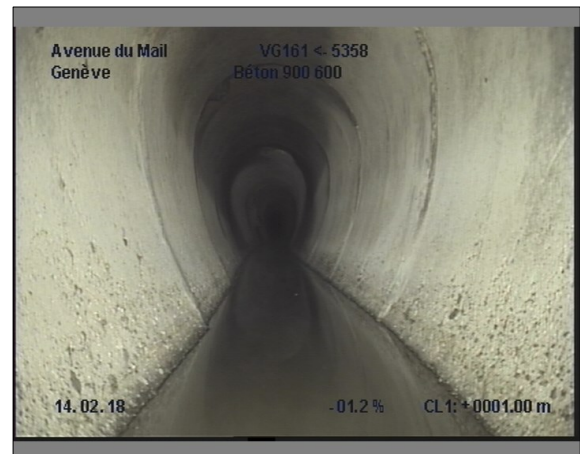
Photo: 15_15_132_A.JPG, 00:00:40 1m, Contre-pente ou flache
