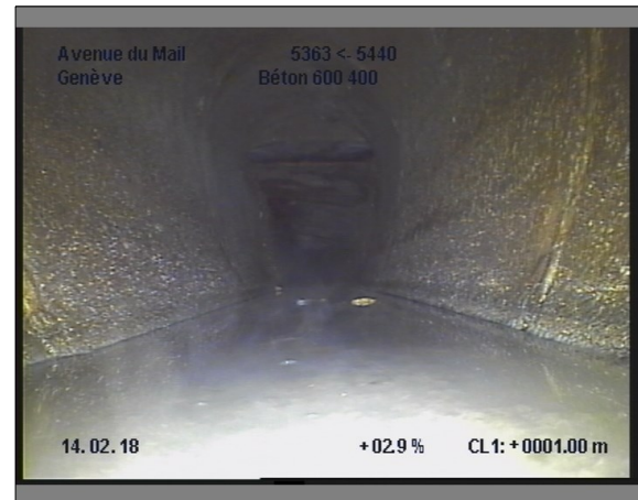
Photo: 26_26_245_A.JPG, 00:00:13 1m, Retenue d'eau
