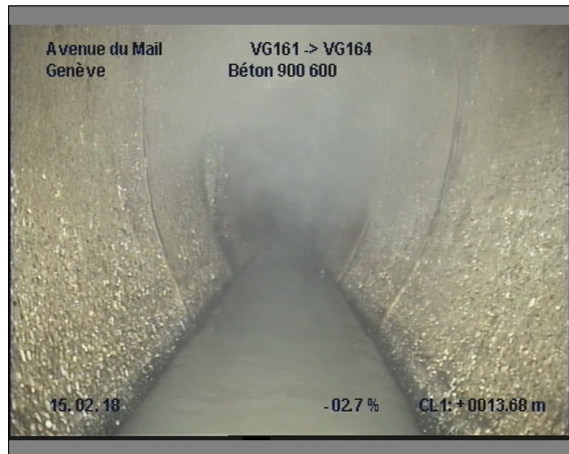
Photo: 14_14_261_A.JPG, 00:01:49 13.6m, Contre-pente ou flache
