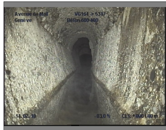
Photo: 9_9_61_A.JPG, 00:00:23 1m, Retenue d'eau
