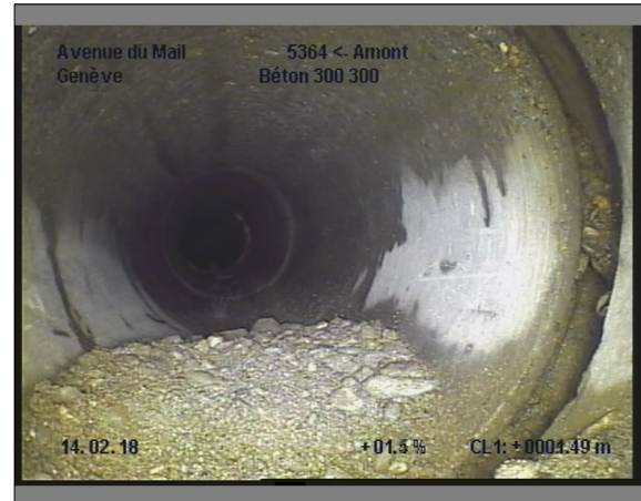
Photo: 24_24_220_A.JPG, 00:00:47 1.4m, Raccord ouvert
