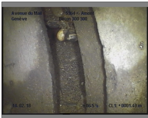
Photo: 24_24_220_B.JPG, 00:00:47 1.4m, Raccord ouvert
