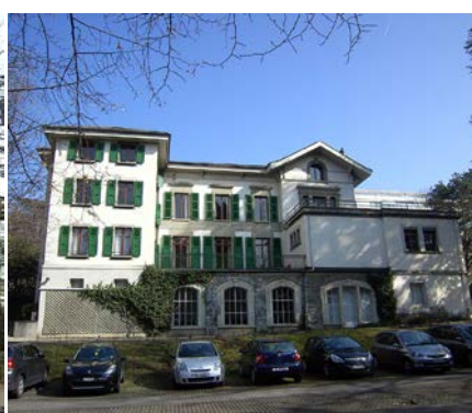
Façade villa Thury, chemin Thury 6
